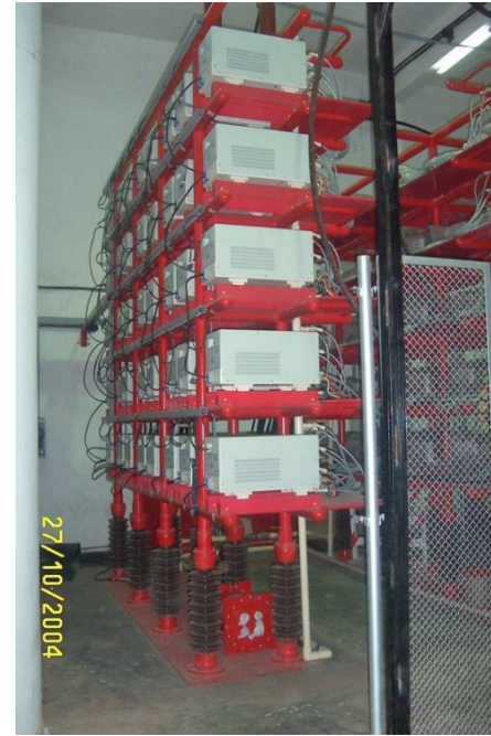
Switched Power Modules on HV Rack
